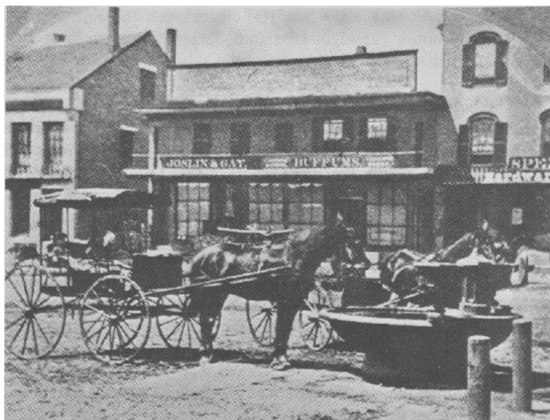
Watering trough and drinking fountain erected 1870 against background of the old Buffum Block
