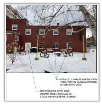
Figure 4. Proposed garage door and windows to be replaced
