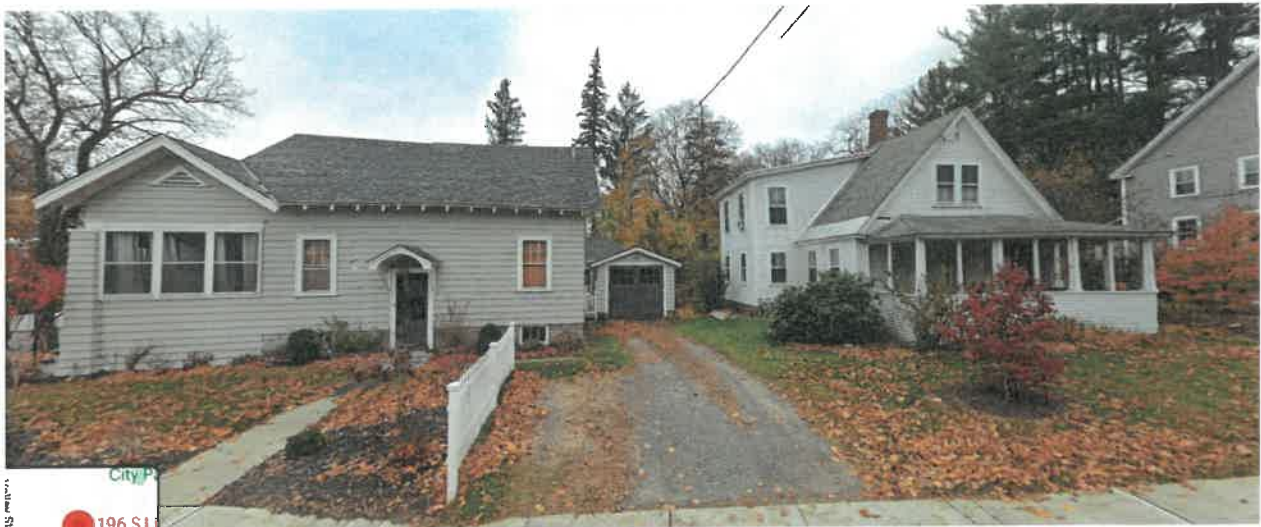
Fig 5. Subject property on left (prior to dormer addition) view from Water street; Existing open porch structure on neighboring residence
