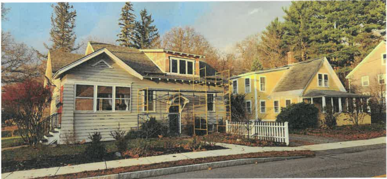
Fig 1. Subject property with Dormer addition under construction showing side entrance
