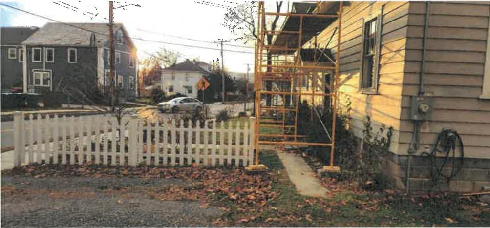
Fig 3. Subject property showing footpath from driveway to side door
