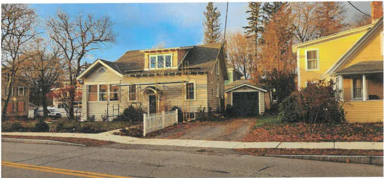
Fig 2. Subject property with Dormer addition under construction showing driveway and garage
