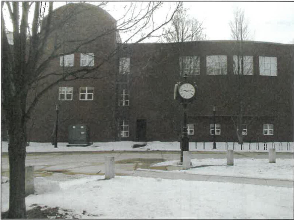
Photograph 11 – Adjacent property, facing west.
