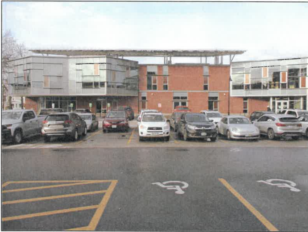
Photograph 5 – Adjacent property, facing north.
