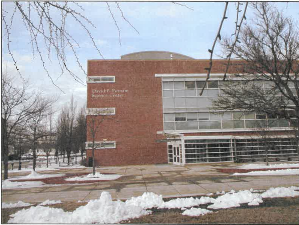
Photograph 1 – Subject property, facing north.
