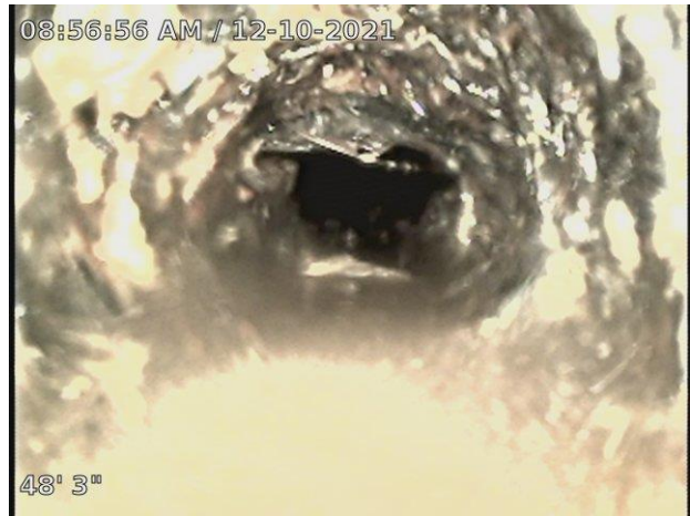
Interior of Pipe
