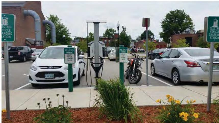
EV charging stations, like the ones pictured above at the Commercial Street parking lot in Keene,<sup>58</sup> will be more cost effective to install if new construction is designed to accommodate future installation by taking steps such as installing all necessary electrical infrastructure, pulling conduit and wire to the appropriate locations, and ensuring concrete work accommodates mounting of charging stations.
