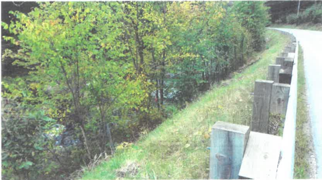
18" RCP Outlet Area – Southern Bank of The Branch
