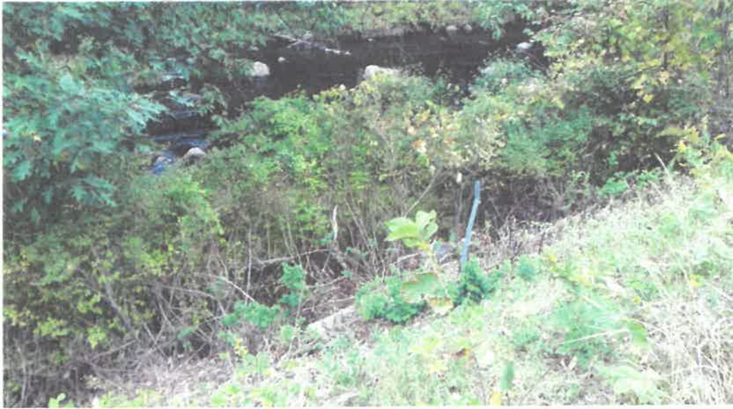
15" RCP Outlet Area – Southern Bank of The Branch
