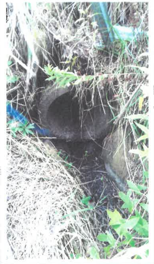
15" RCP Outlet – Southern Bank of The Branch
