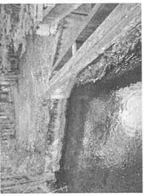
Upstream Training Wall, Left Abutment
