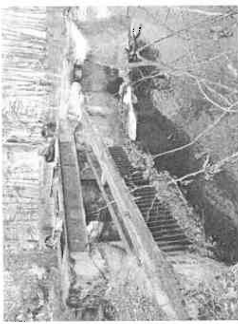
Diversion Intake Structure
