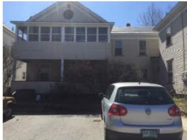
57 Dunbar Street 5-Unit used as 4-Unit, 8,712 SF Lot
