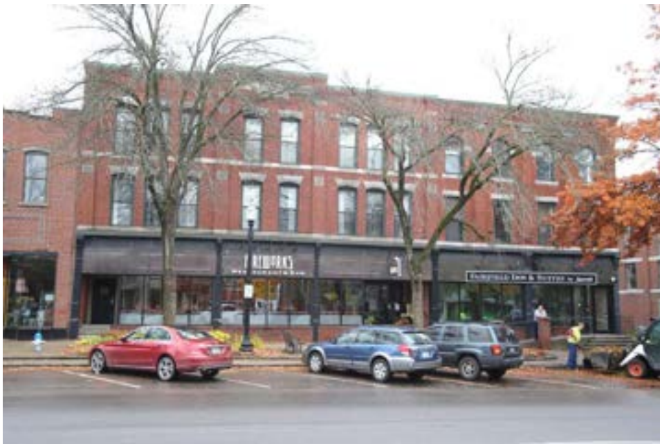
Photo 58) 1891 3-Story Block, 22-30 Main Street (575-054) Reference: IMG_9755
