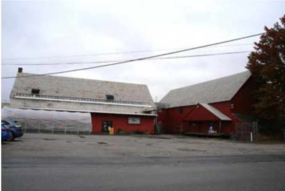
Photo 37) 1875 Brick Building and Barn, 24-40 Dunbar Street (585-001) Reference: IMG_9714
