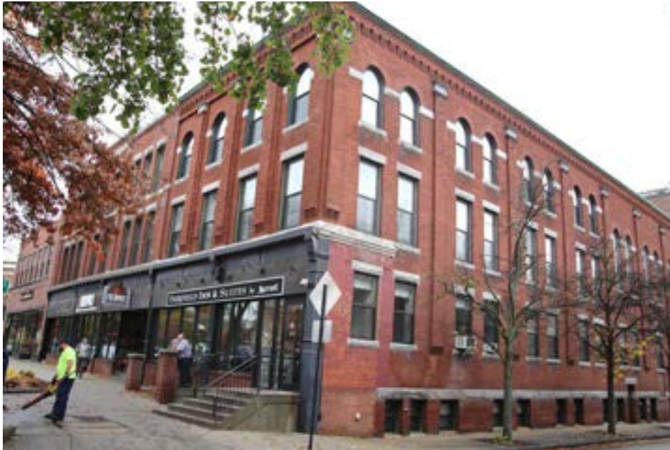
Photo 59) 1891 3-Story Block, 22-30 Main St. (575-054) at Church St. Intersection Direction: N Reference: IMG_9754
