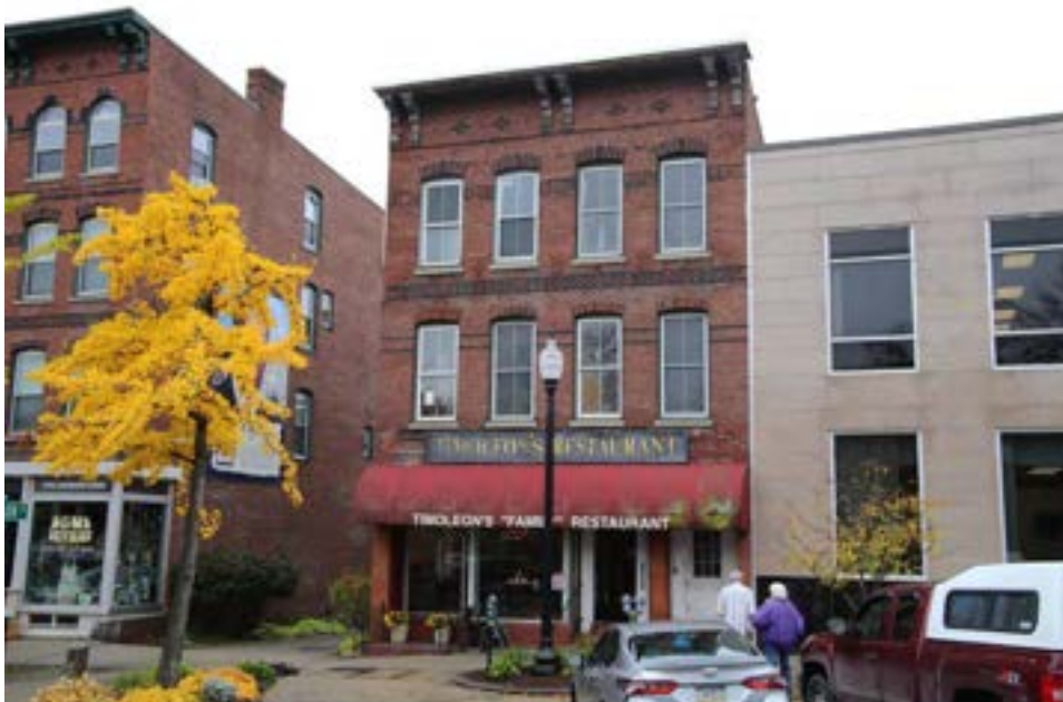
Photo 60) 1900 3-Story Building, 27 Main Street (575-029) Reference: IMG_9676
