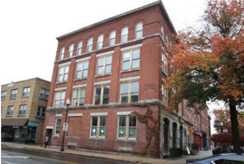
Photo 11) 1900 4-Story Brick Block, 50 Central Square (575-051), View from West St. Direction: NW Reference: IMG_9656
