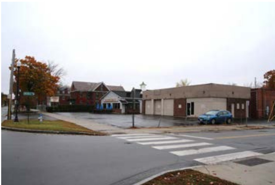
Photo 86) 1950 1-Story Brick & Concrete Garage, 125 Main Street (584-063) Reference: IMG_9690
