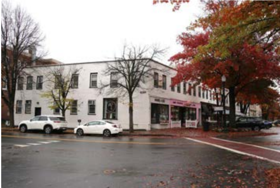
Photo 7) 1900 2-Story Brick Block, 32 Central Square (568-061) Reference: IMG_9648
