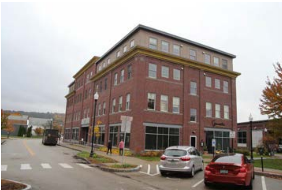
Photo 101) 2009 4-Story Brick Building, 51 Railroad Street #A (574-041-000-00A) Reference: IMG_9741
