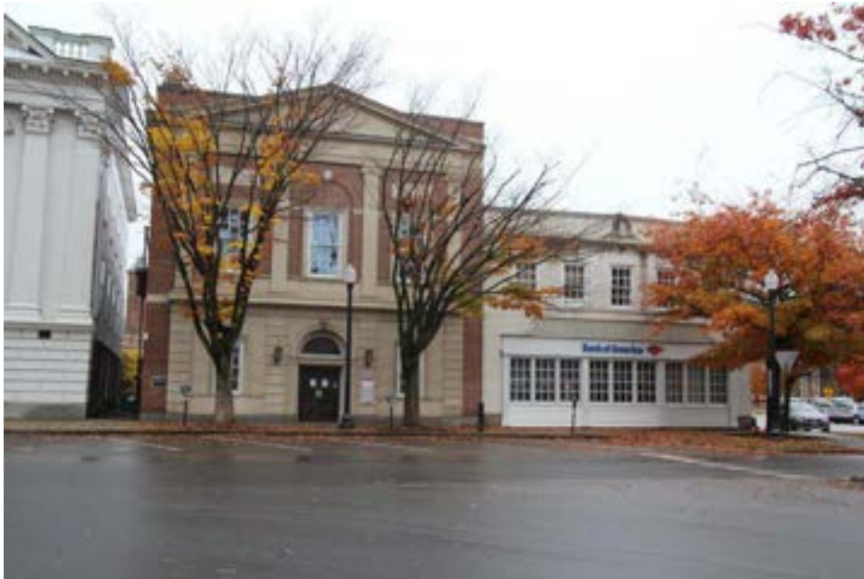
Photo 4) 1926 2-Story Block, 20 Central Square (568-063)
