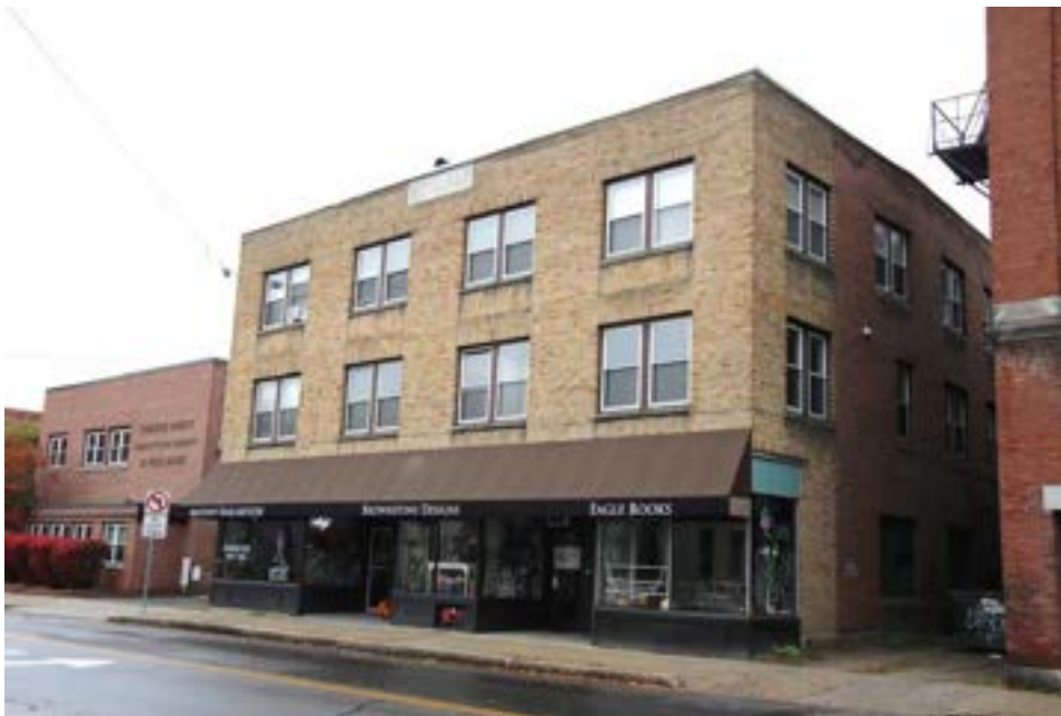
Photo 120) 1927 Howe Building, 19-25 West Street (575-050) Reference: IMG_9657
