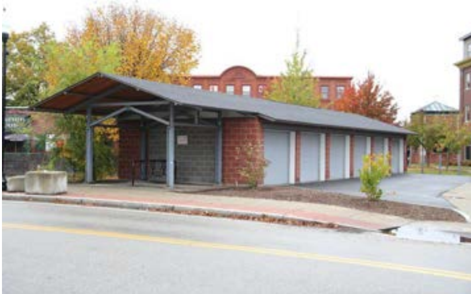
Photo 31) Storage Unit, Cypress Street (574-041) Reference: IMG_9734
