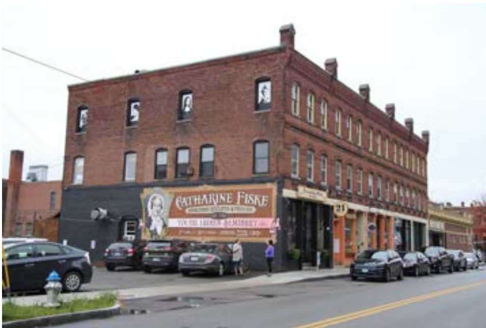
Photo 55) 2-20 Main St. rear elevation (575-053), View from Roxbury St. Reference: IMG_9764
