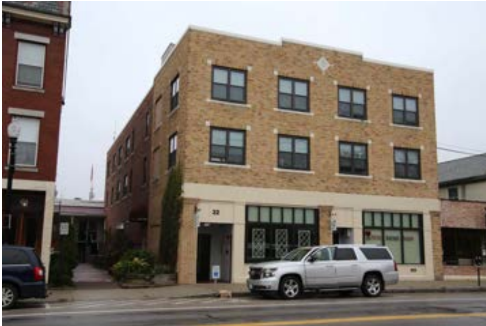
Photo 113) 1910 3-Story Building, 32-34 Washington Street (568-065) Reference: IMG_9626
