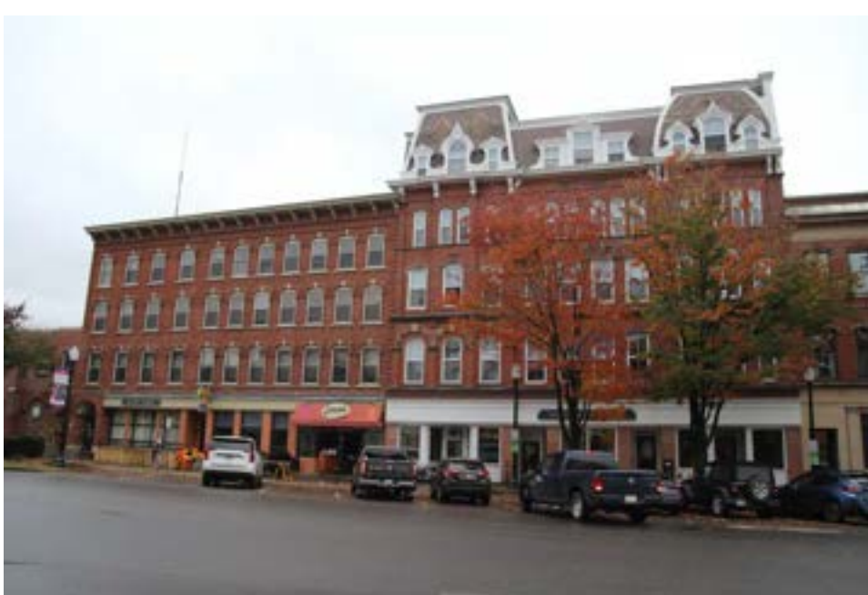
Photo 2) 1870 Colony's Block, 4-7 Central Sq. (at right) (568-074) 1900 City Hall, 3 Washington St. (at left) (568-073) Reference: IMG_9766
