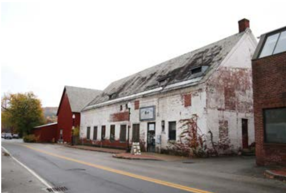
Photo 38) 1875 Buildings, 24-40 Dunbar Street (585-001), View from Eagle Ct. Reference: IMG_9719
