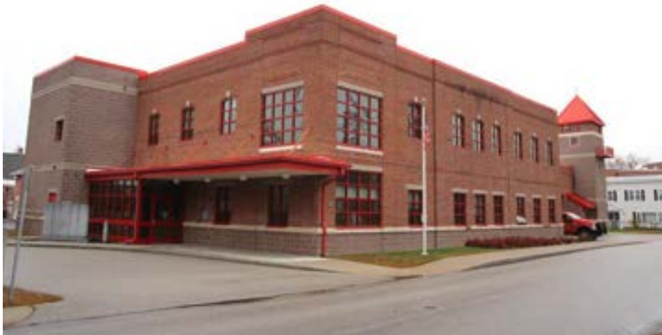
Photo 106) 2012 Fire Station, 31 Vernon Street (548-051) Reference: IMG_9637
