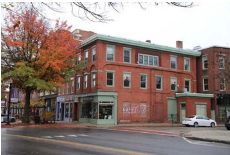
Photo 8) 1890 3-Story Brick Block, 37 Central Square (568-003) Reference: IMG_9645
