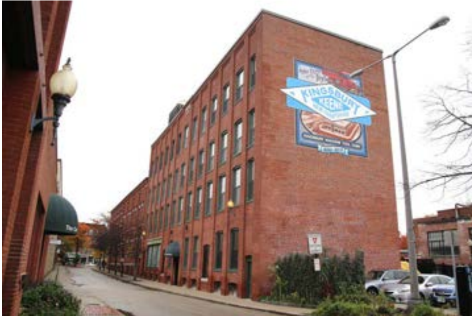
Photo 19) 1900 Gurnsey's 4-Story Brick Block, 16 Church Street (574-007) Reference: IMG_9752
