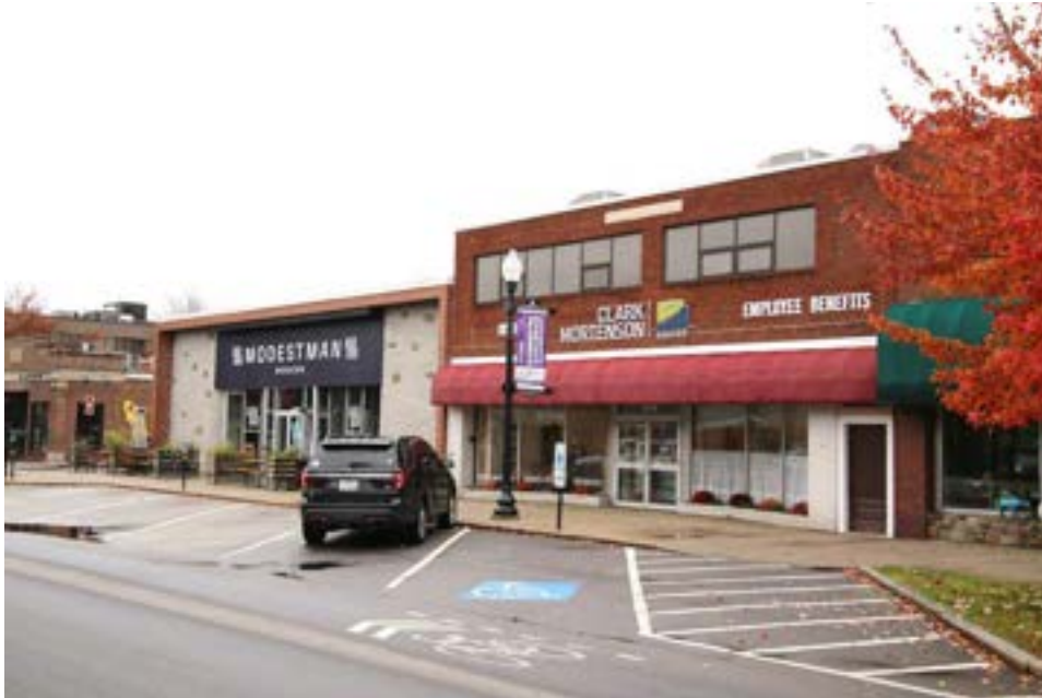
Photo 77) 1930 1-Story Brick Block, 100 Main Street (at left) (575-059) 1930 Whipple-MaLaughlin Block, 102 Main Street (at right) (575-060) Reference: IMG_9727
