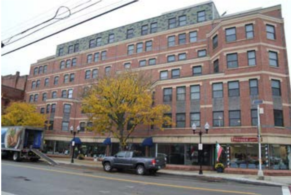
Photo 3) 1983 Colony's Block rear addition (south elevation), 4-7 Central Sq. (568-074), View from Roxbury St.
