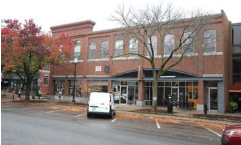
Photo 63) 1920 2-Story Block, 42-46 Main Street (575-055) Reference: IMG_9748
