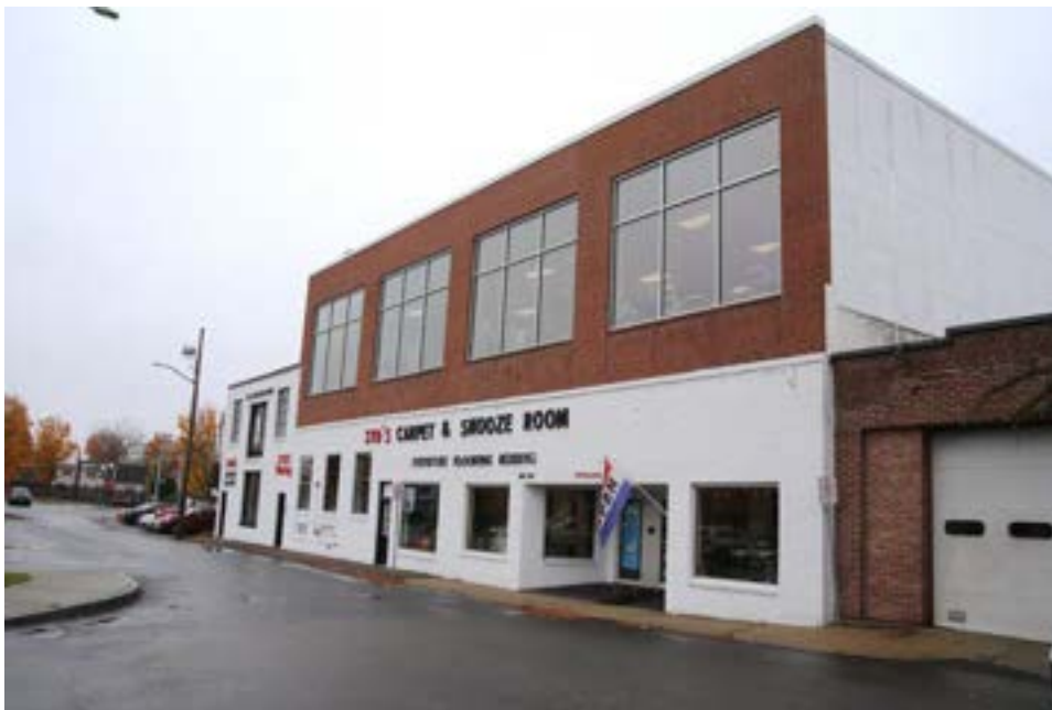
Photo 104) 1940 2-Story Brick Building, 43 St. James Street (575-036) Reference: IMG_9668
