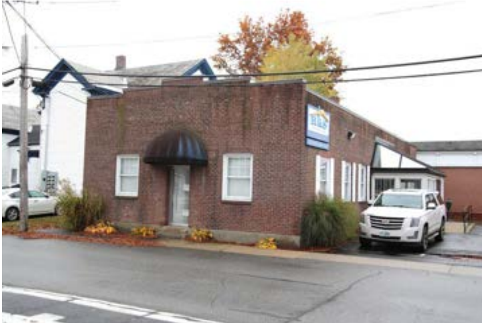
Photo 35) 1850 1-Story Brick Building, 17 Dunbar Street (585-014) Reference: IMG_9712
