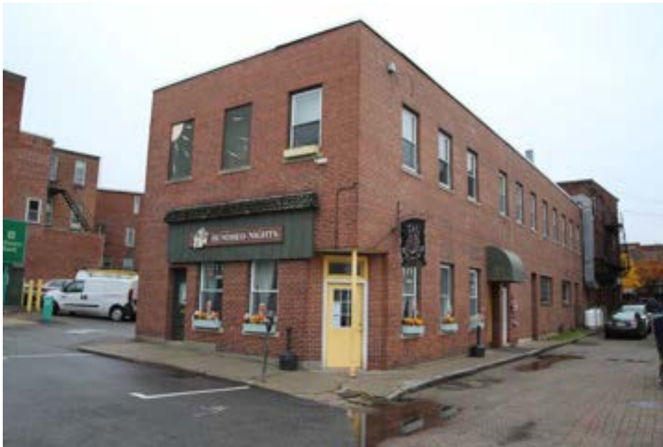
Photo 61) 27 Main St. rear elevation (575-029), at Lamson/Federal St. Intersection Reference: IMG_9666
