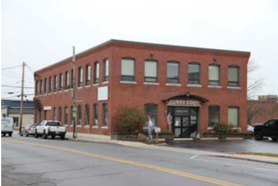
Photo 43) 1880 2-Story Brick Building, 7 Emerald St. #101 (575-005-000-001) Direction: NW Reference: IMG_9692
