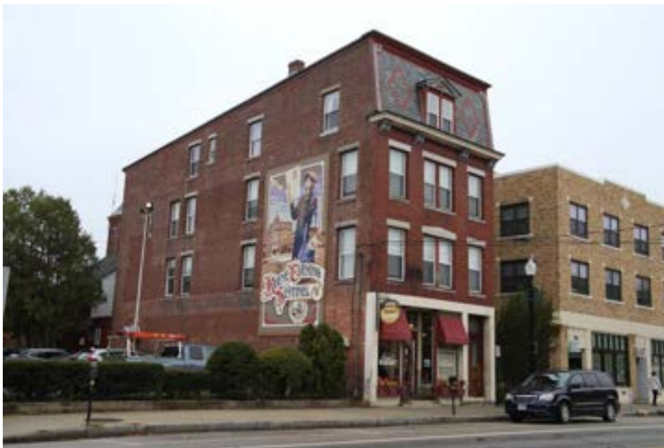
Photo 110) 1900 4-Story Brick Building, 26 Washington Street (568-064) Reference: IMG_9624
