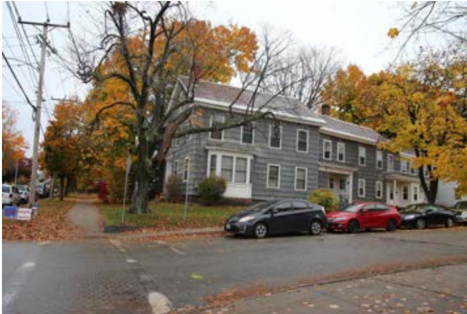
Photo 117) 1900 Residence, 57 Washington Street (569-014), at Spring St. Intersection Reference: IMG_9631
