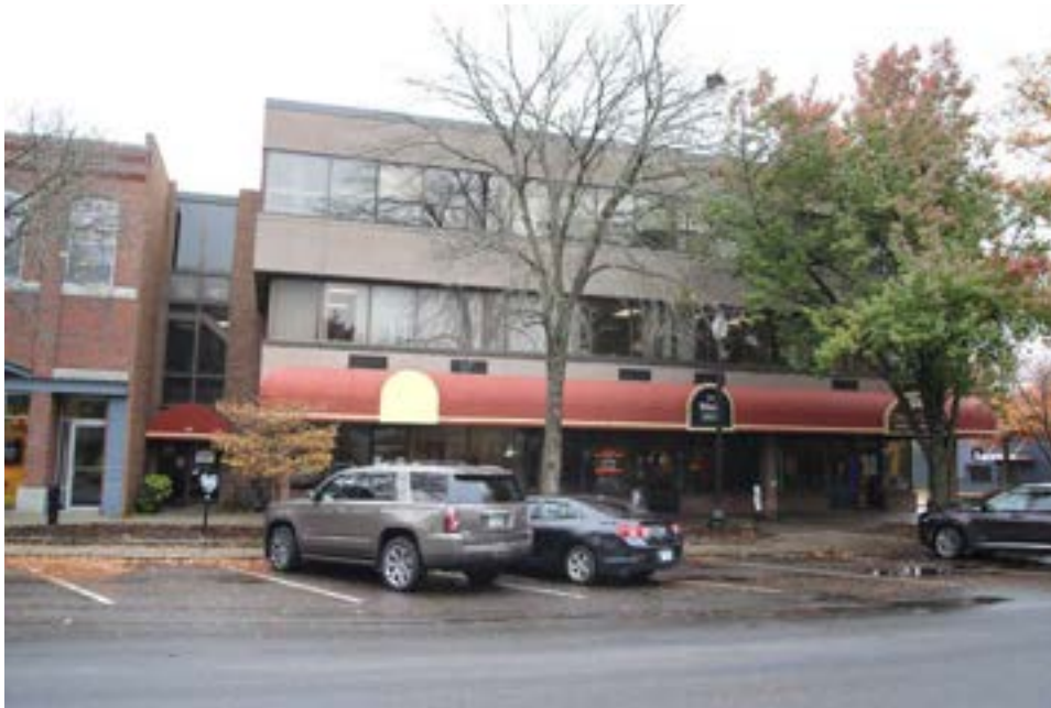
Photo 67) 1930 3-Story Building, 64 Main Street (575-056) Reference: IMG_9747
