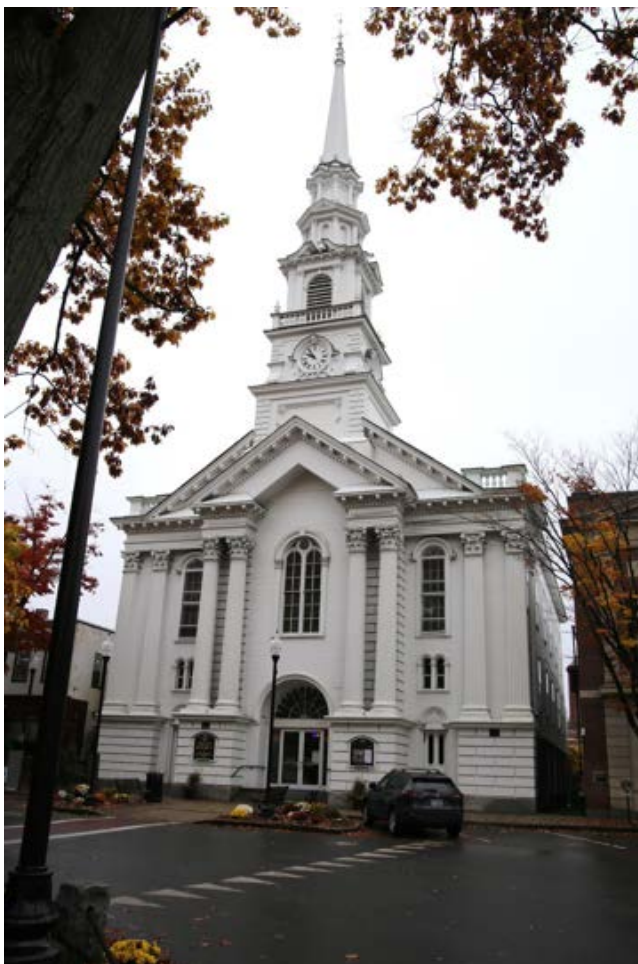
Photo 6) 1786 United Church of Christ, 23 Central Square (568-062) Direction: N Reference: IMG_9651
