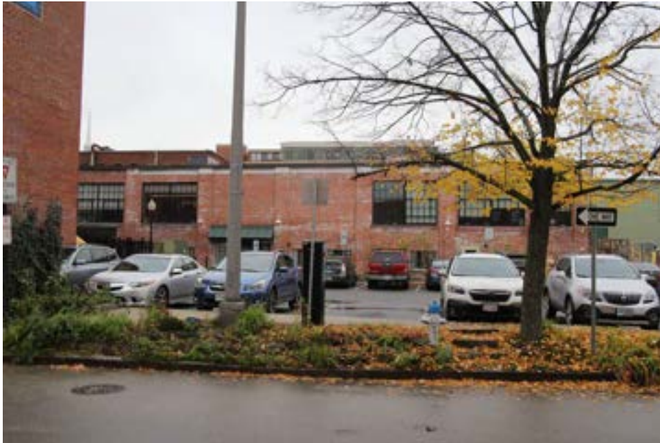
Photo 103) 1910 Blaisdell Building, 25 Roxbury Street, view from Church St. Reference: IMG_9753
