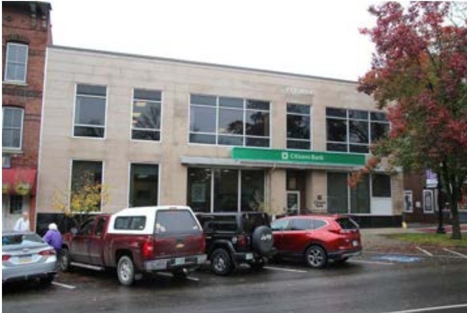
Photo 57) 1900 2-Story Building, 15 Main Street (575-030) Reference: IMG_9675
