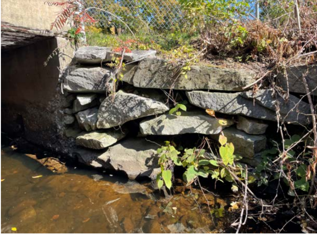
Stone retaining wall at southeast corner, looking northeast
