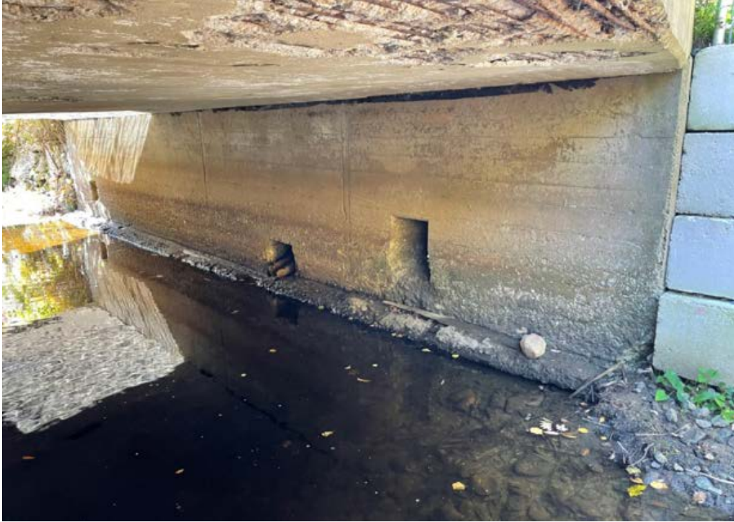
Western bridge abutment, looking southwest
