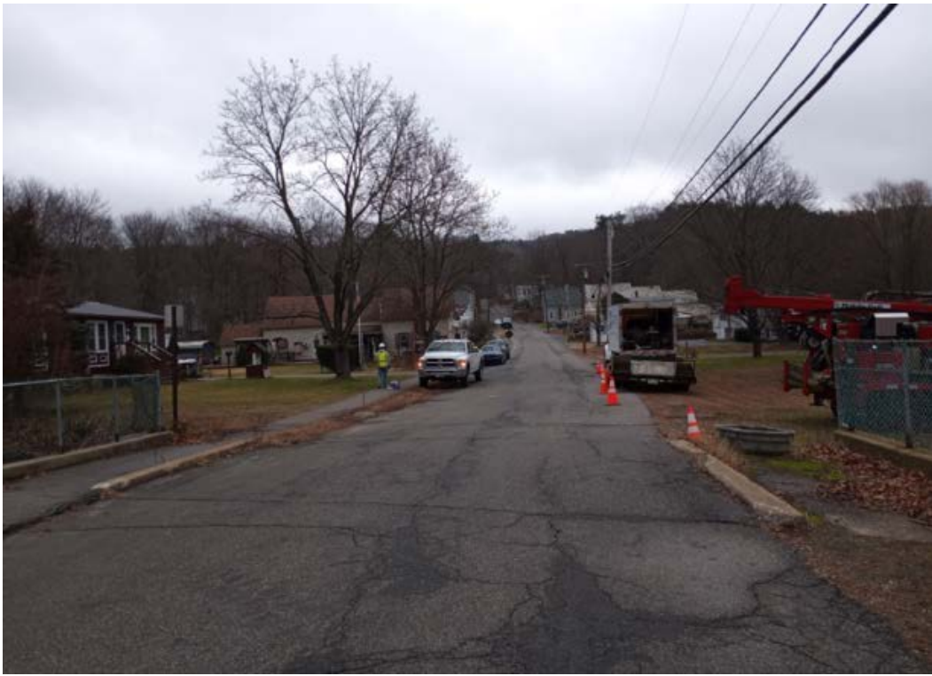
Western side of bridge site, looking east
