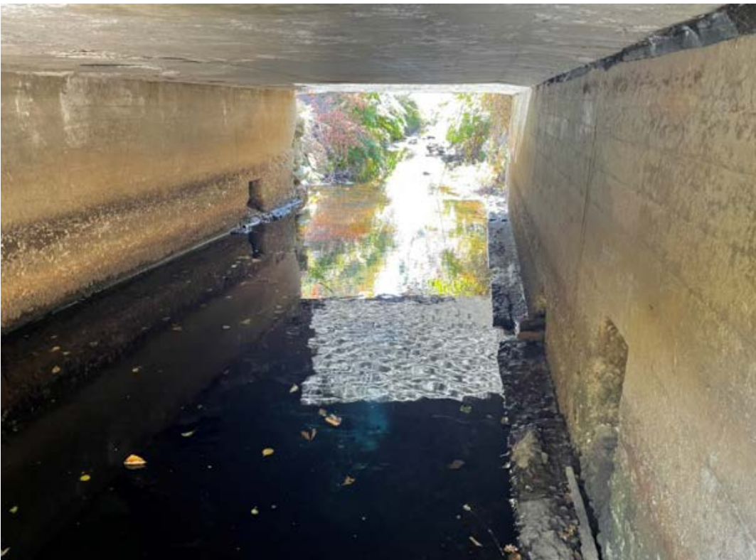
Under the bridge, looking south
