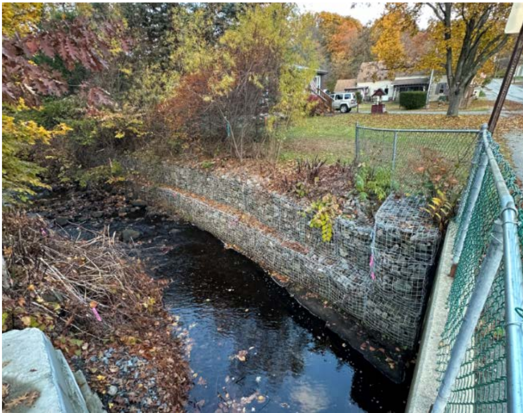
Gabion basket stabilization at northeast corner of bridge
