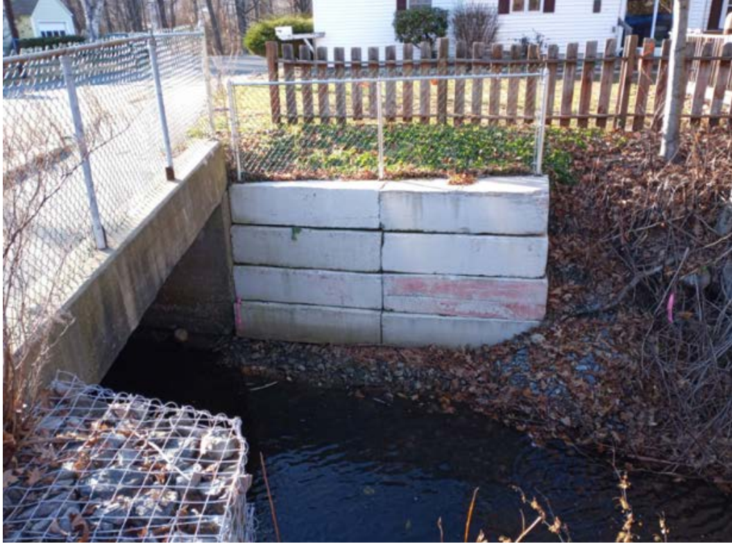
Temporary stream bank stabilization at northwest corner of bridge
