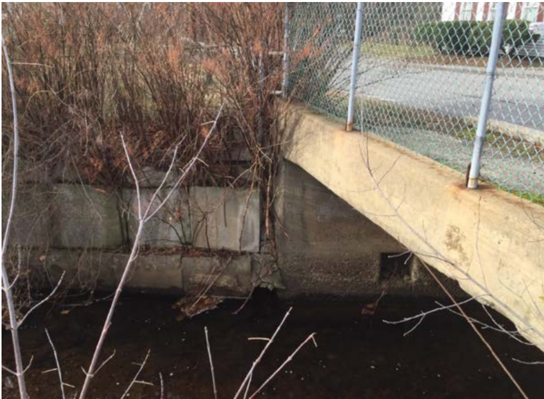
Stone / concrete retaining wall at southwest corner, looking west
