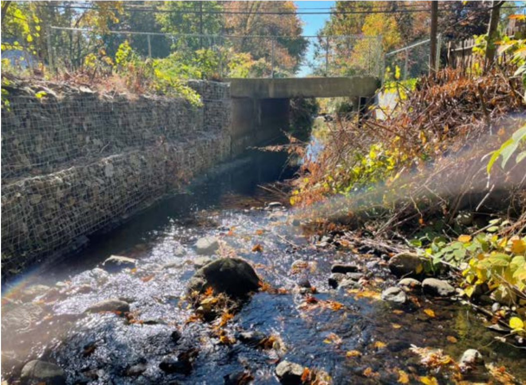
Beaver Brook, upstream of bridge, looking south
