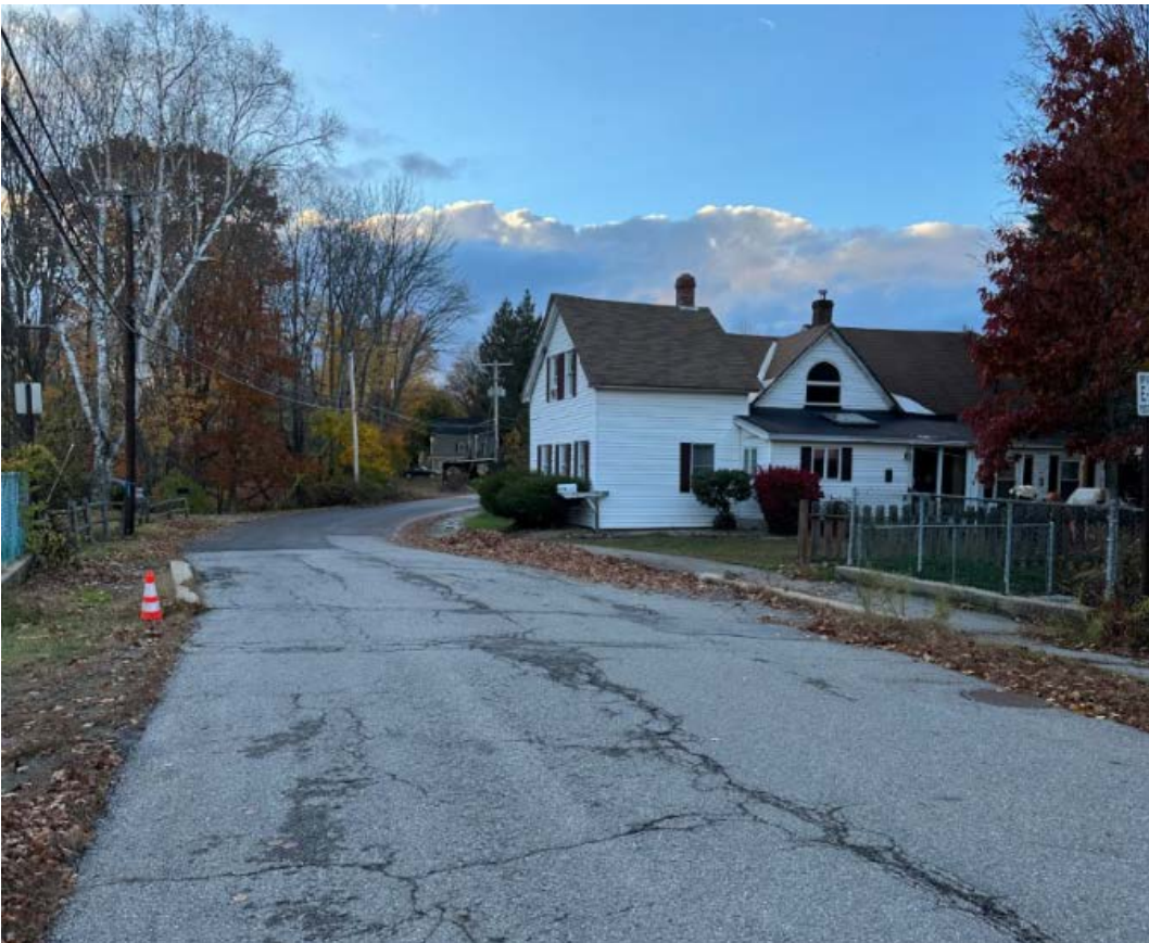
Eastern side of bridge site, looking west
